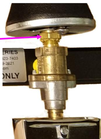
4. An efficient flame is mostly blue with a slight orange tip. Once the flame is large enough, stop loosening and use the silver disk on the air mixer to adjust. Do this on all 3 control valves. Then you're ready to use!
